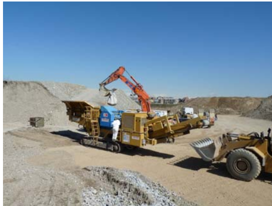
Fig. 1. The mobile plant
