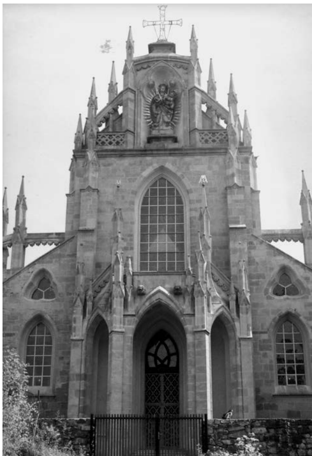
Fig. 13. Façade of the cloister church of the Assumption and Saint Benedictine and Wolfgang in Kladruby (photo: O. Czerner)
