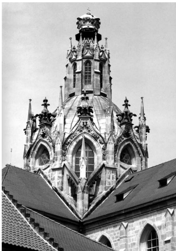
Fig. 14. Façade of the cloister church of the Assumption and Saint Benedictine and Wolfgang in Kladruby (photo: O. Czerner)
