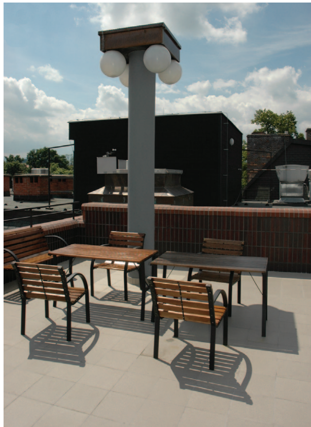
Fig. 10. Terrace on the highest floor of the building, +13,00 (photo: P. Amałowicz)
