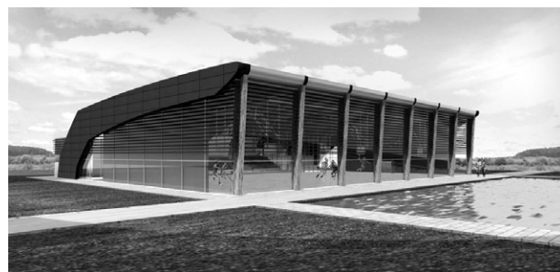
Fig. 1 Front view of the sports hall
