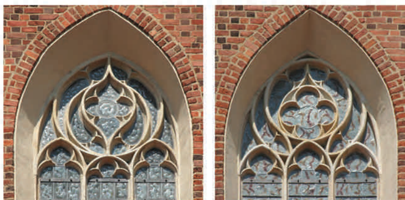
East windows of the south façades
