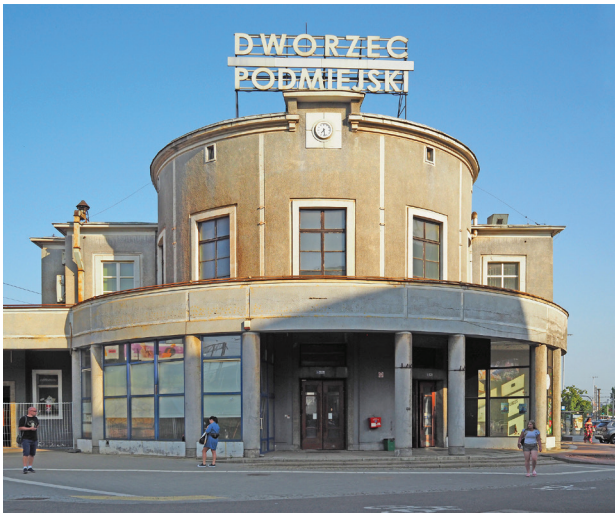
Fig. 4. Front elevation (south-east) of the Gdynia Główna Suburban Railway Station, June 2022 (before the start of restoration works) (photo by A. Orchowska-Smolińska)
