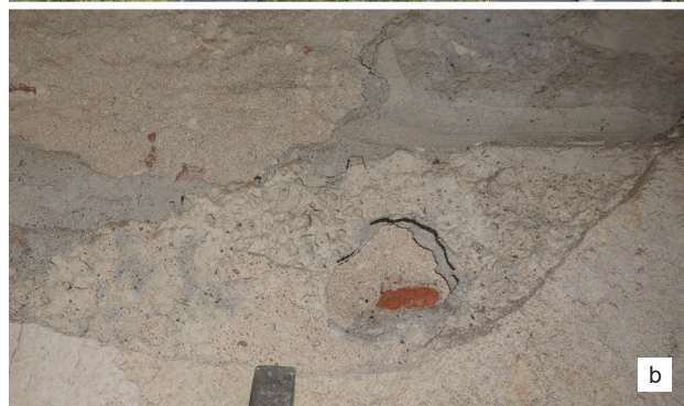
Fig. 9. Solutions characteristic of the fifth phase: a) the façade of the kitchen tower from the second stage of the fifth phase, referring in detail to the façade from the fourth phase (there are no traces in the homogeneous wall suggesting the later addition of neo-Gothic dormers), b) a well-preserved fragment of unpainted plaster with a rustication profile, used on the tower and the side and rear façades of the nave (the alcoves were prepared in the same way using lighter plaster) (photo by S. Bakalarczyk, 2023)
