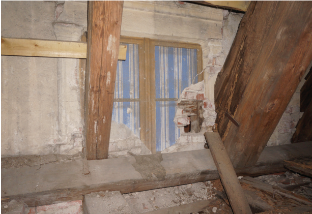
Fig. 8. The gable wall of the western wing, built as part of the first stage of the fifth phase. The brick and skeleton structure of the gable is visible, also repeated in the knee walls (photo by S. Bakalarczyk, 2023)
