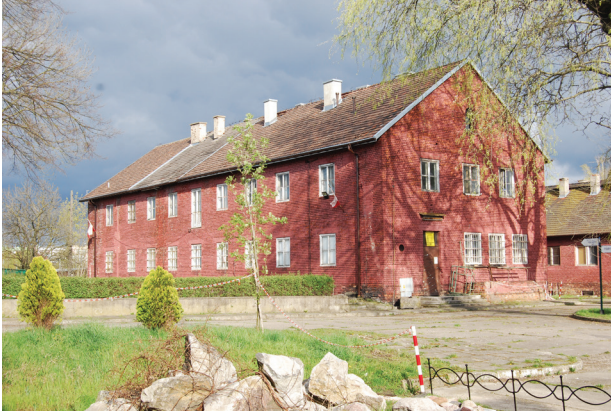
Fig. 4. Office and accommodation building (photo by P. Mierosławski)
