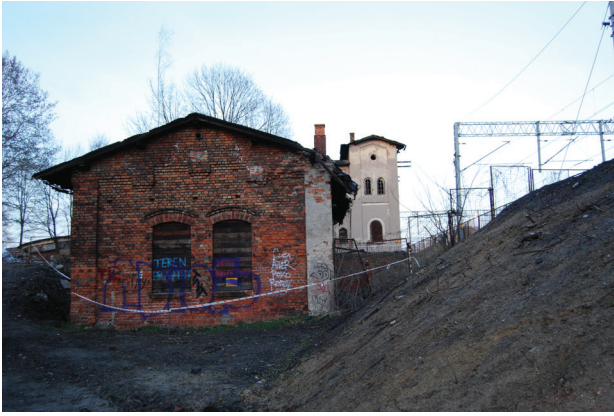
Fig. 8. Pumping station (photo by P. Mierosławski)
