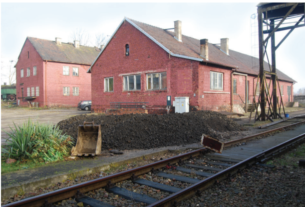
Fig. 5. Office and warehouse building (photo by P. Mierosławski)
