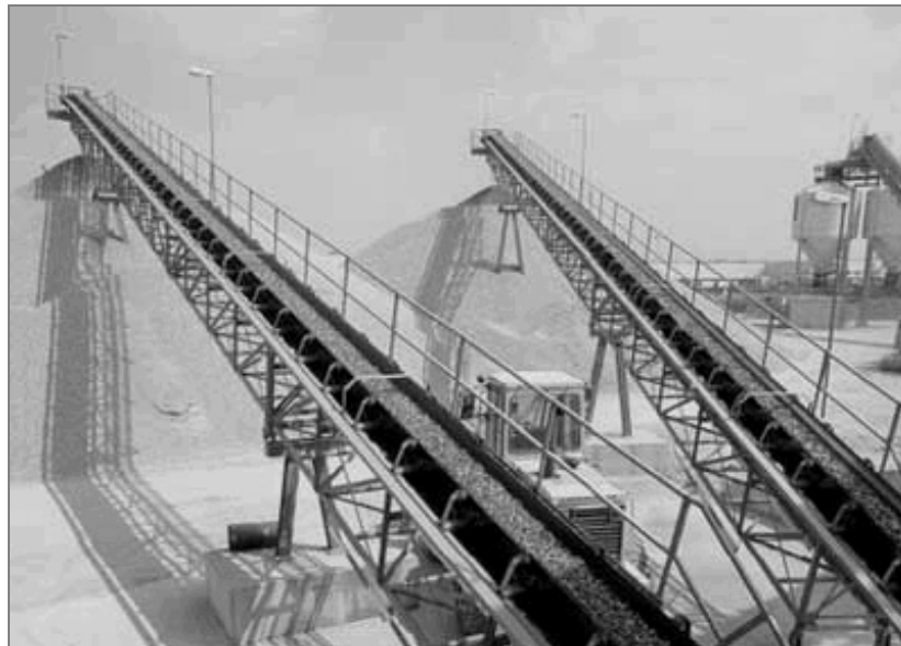
Fig. 1. A typical belt conveyor structure used for in-factory transport [9]
