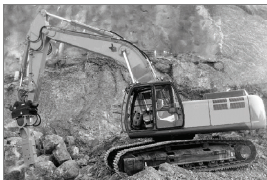
Fig. 1. Crawler excavator in operation
