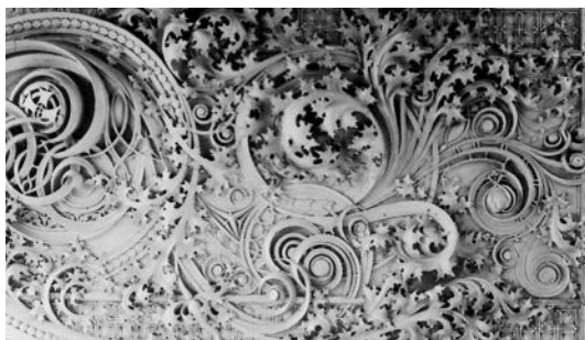
Ryc. 104. Ornament żelazny, odlewany - detal z budynku Schlesinger and Mayer Department Store w Chicago – arch. L. Sullivan (1904) Fig. 104. Iron, molded ornament – detail from Schlesinger and Mayer Department Store in Chicago, arch. L. Sullivan (1904)
