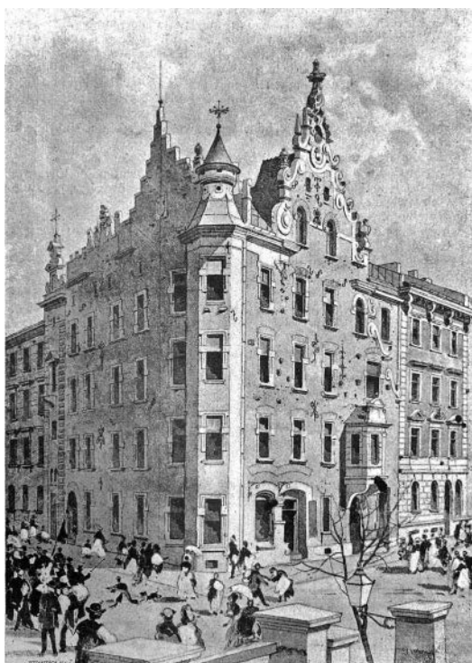
Ryc. 1. Dom Pod Pajakiem , wg. akwareli St. Tondosa 1890 Fig. 1. The house Under the Spider , watercolour by St. Tondos 1890
