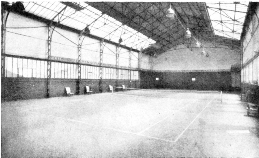
Abb. 133. Tennishalle Montparnasse, Paris
