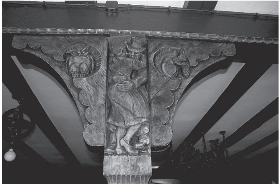
Fig. 10. “Andrzejówka” shelter. Cap of the column with the motif of a dancing couple. Photo by author, 2008
