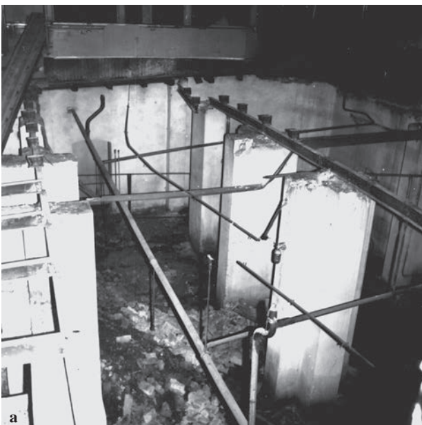
Fig. 2. Replacement of floor construction in 1980: a) view of disassembled floor construction; b) floor construction metal I beams
