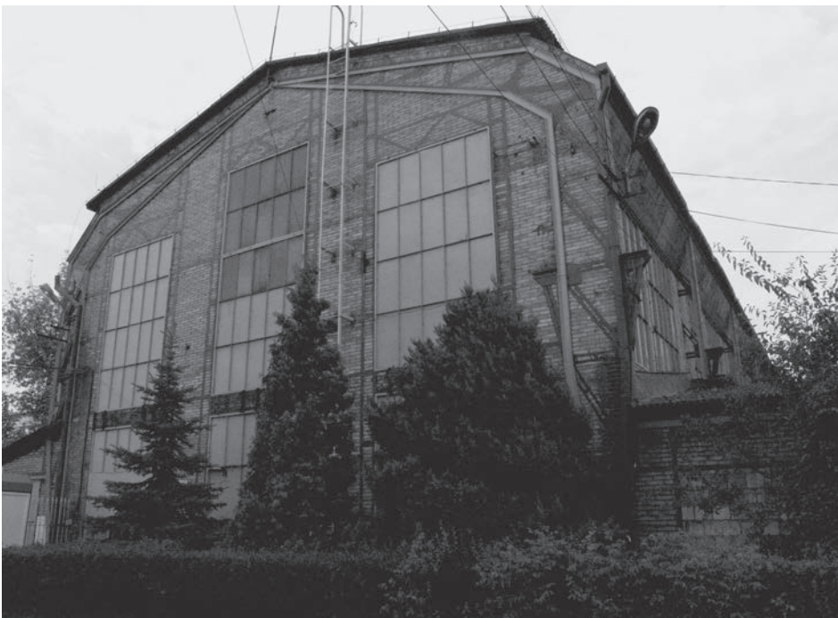
Fig. 2. Starachowice, factory of ammunition. Photo by author, 2009
