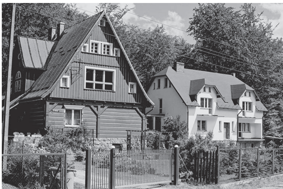
Fig. 4. Georg Wichmann House in Michałowice. Photo by author, 2001.
