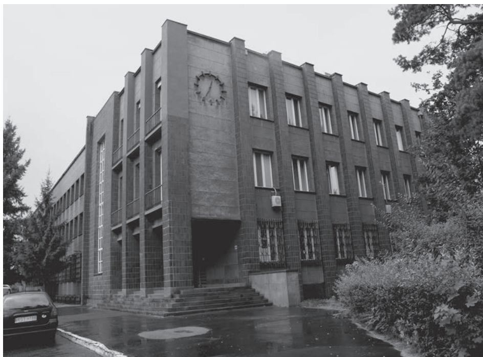
Fig. 3. Stalowa Wola, the management building. Photo by author, 2009
