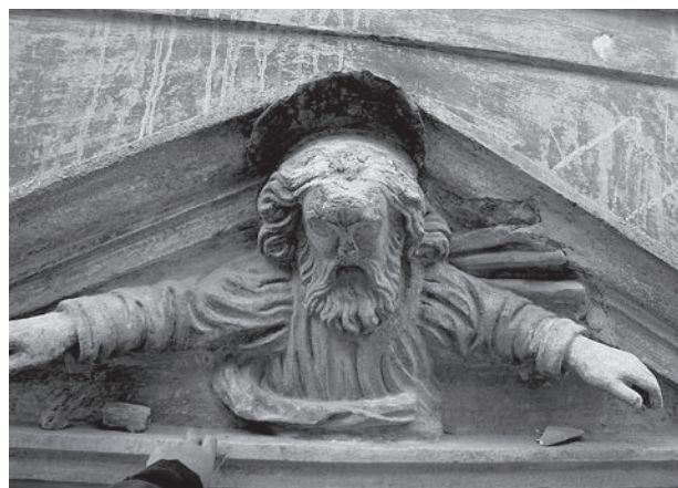
Fig. 14. Scholtz-Wolfowitz house. Sculpture of God the Father on the pediments above outermost windows of the third floor
