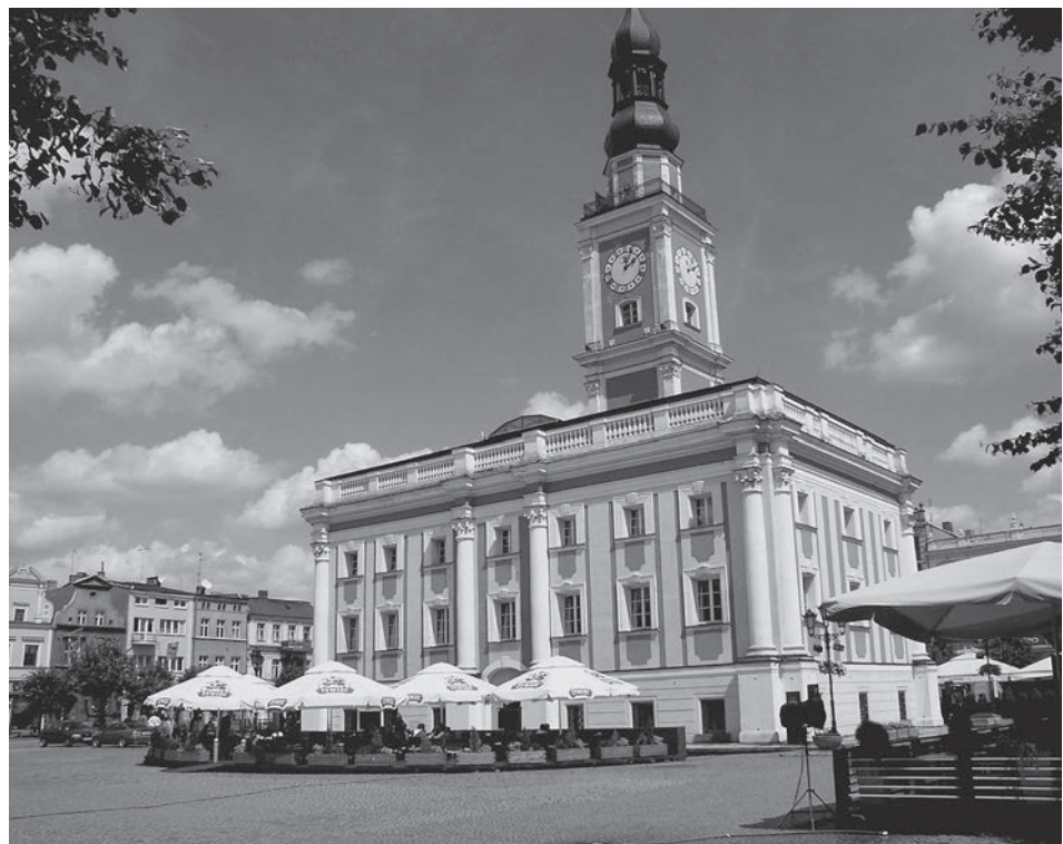
Fig. 1. View of Town Hall in Leszno located on the Market Square
