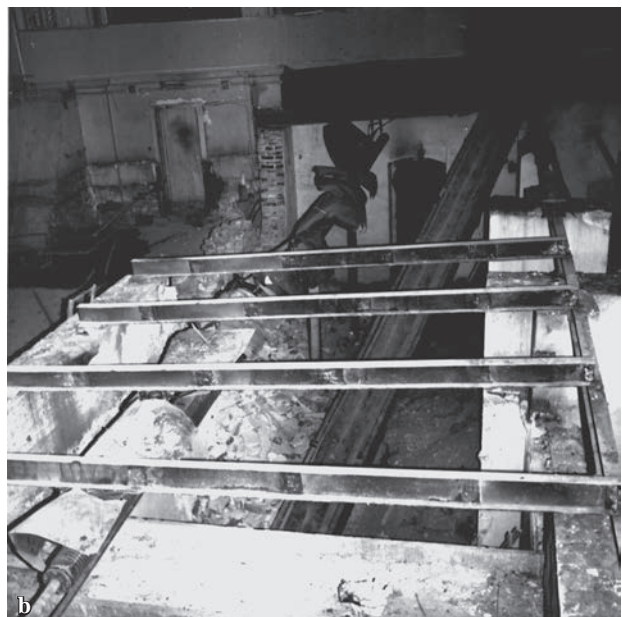
Fig. 2. Replacement of floor construction in 1980: a) view of disassembled floor construction; b) floor construction metal I beams
