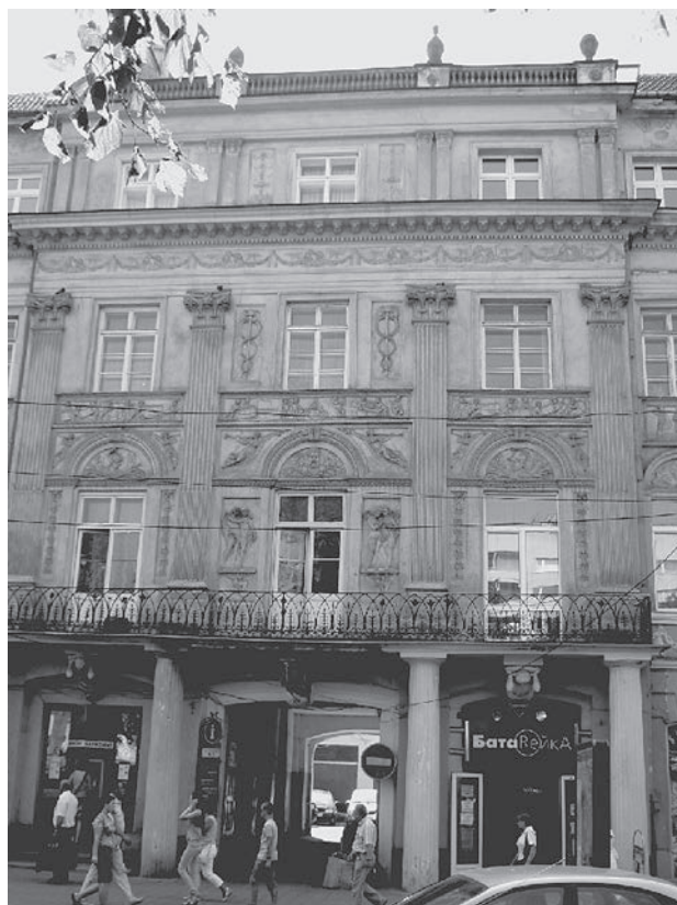
Fig. 5. The Hausner house in prospect Svobody 1–3 (1810–1811, 1829–1822)
