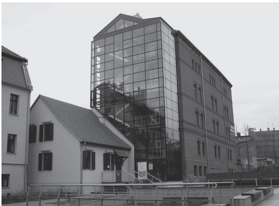
Fig. 10. New cubature view with a staircase and person elevator added to the old steam mill on Mill Island in Bydgoszcz. Photo by M. Rusnak, 2010
