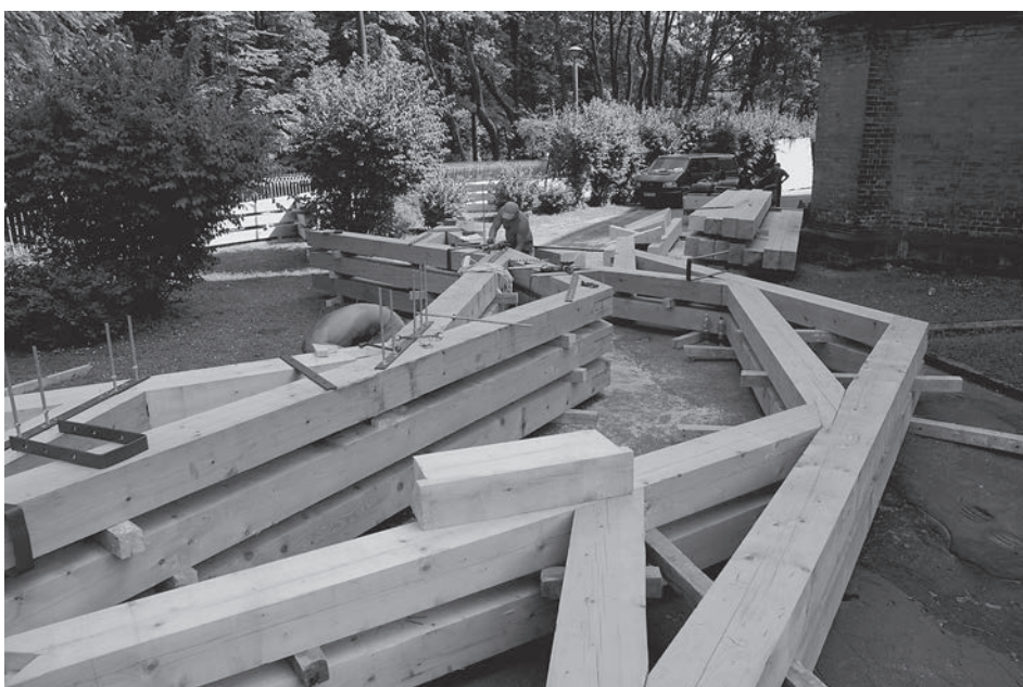
Fig. 2. Execution of the reconstructed roof framing trusses
