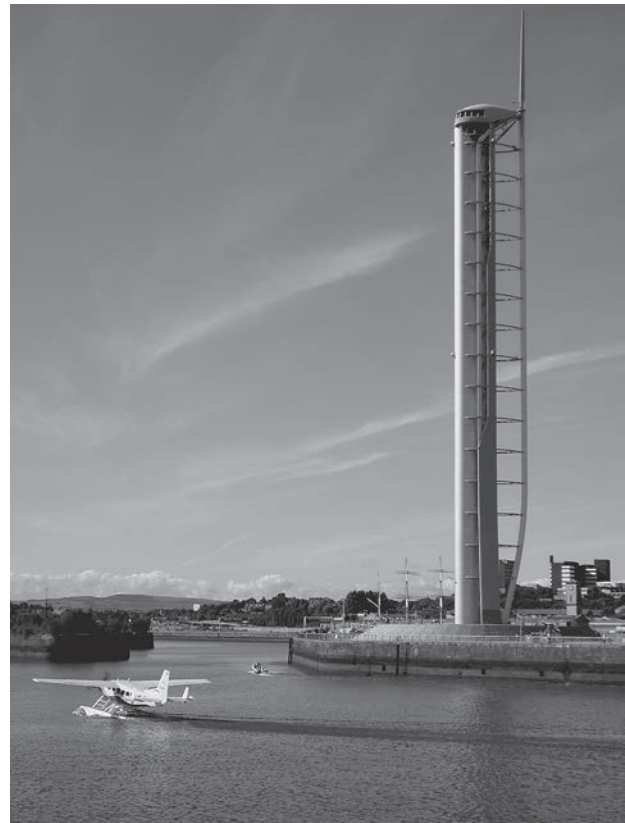
Fig. 2. Glasgow Tower – in Glasgow Science Center, designed by Richard Horden. Photo by J. Woźniak
