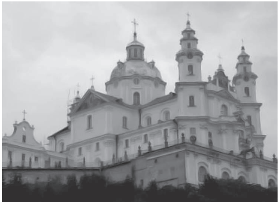
Fig. 1. St. Uspenska Lavra in Pochaiv. Overall view
