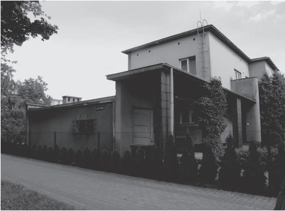
Fig. 14. Stalowa Wola, the building complex of the Management Colony (1937–1939). Photo by author, 2010
