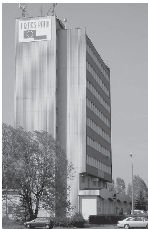
Fig. 8. Office building in Przylep village near Szczecin – condition in 2004. Photo by author
