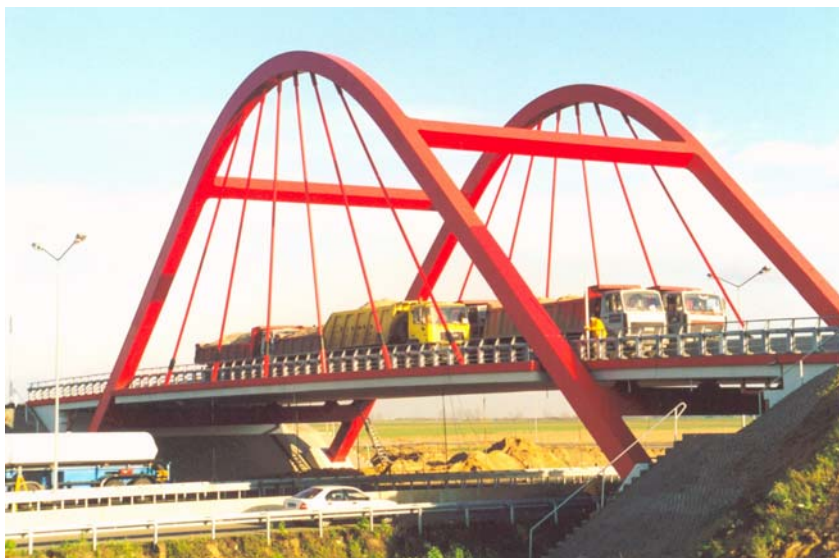
Fig. 4. Arch viaduct A016 over the highway A4 during load tests
