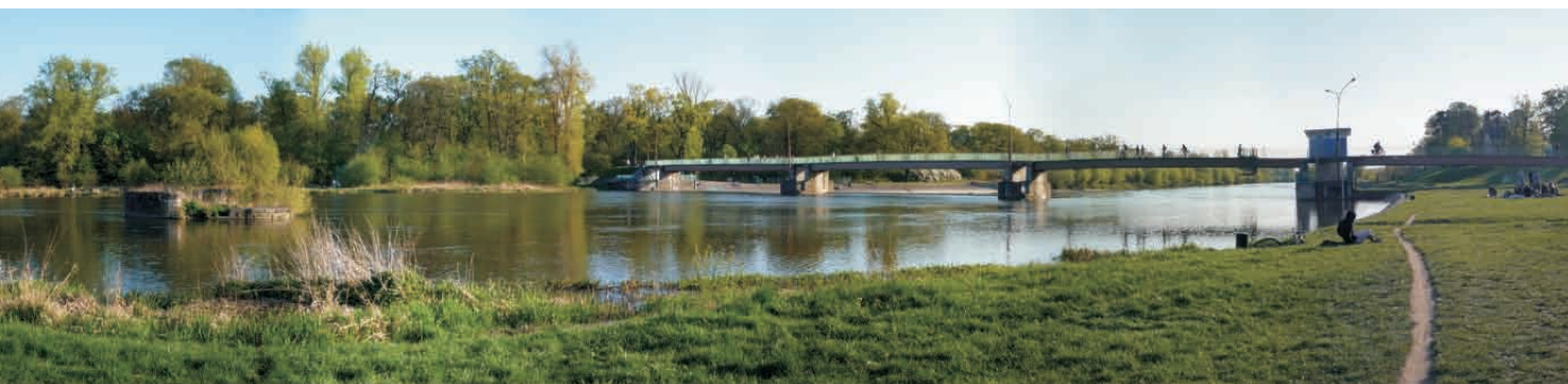
Fig. 3. View of barrage Opatowice
