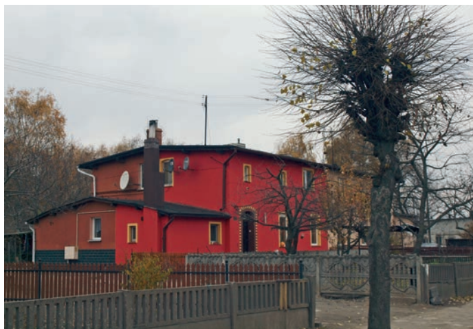
Fig. 7. Babkowice, example of the renovated quadruple house
