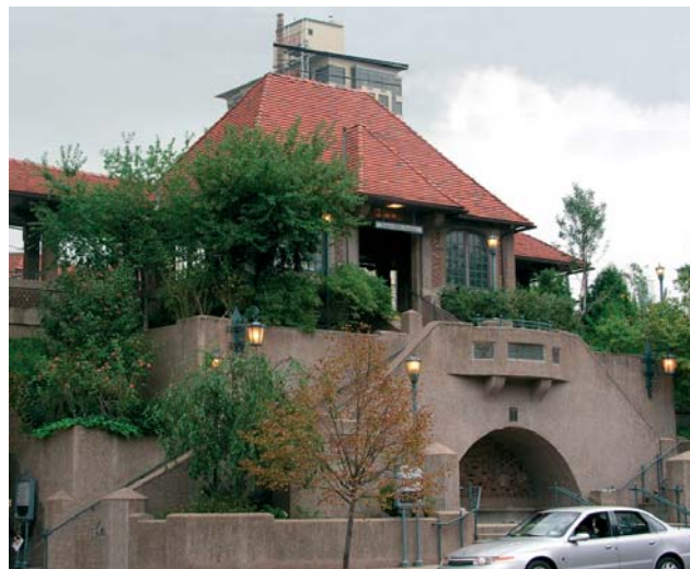
Fig. 9. Subway station Forest Hills (photo by K. Pawłowska)
