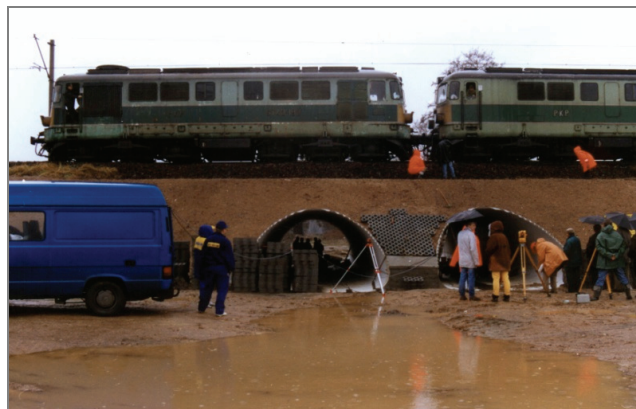
Fig. 9. The passage of two locomotives along the building structure analysed
