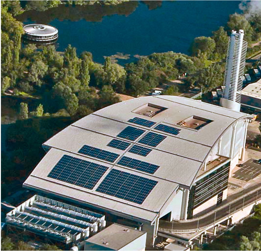
Rys. 5.5. Spalarnia odpadów Lakeside Energy from Waste (Colnbrook, Wielka Brytania) z zainstalowanymi panelami PV [www.ManchesterHistory.net, www.belectric.co.uk]
