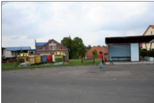
Ryc. 169. Skwer objęty projektem w 2003 r. – widok od strony drogi (jesień 2008) Fig. 169. Square included in the project in 2003 – view from the side of the road (autumn 2008)
